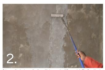
Prime wall prior to application with two coats of Cemcrete's FlexBond/water solution (diluted 1 part FlexBond to 4 parts water). NOTE: For exterior use, replace the FlexBond with CreteBond. Dilution ratios stay the same as for FlexBond.
