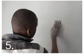
When the first coat of CemCote is dry (but within 24 hours), sand lightly by hand, in a circular motion, with 120 grit Abranet sandpaper.
