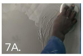
Apply the second coat and any additional coats as needed (max 0.8mm per coat), in the same manner as the first coat, until a smooth finish is achieved. First with a sponge and then...
