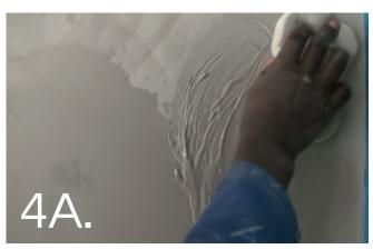
Using a firm sponge rub the first layer thinly onto the surface, follow this method small sections of the wall at a time...
