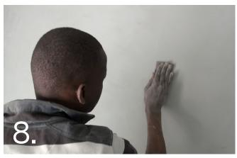
Once the final coat of CemCote is dry (but within 24 hours after the application), sand lightly with 240 grit Abranet sandpaper in a circular motion, to not leave any sanding marks and ridges on the surface.
