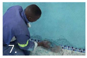
Apply the BeadCrete to the surface with a steel trowel forcing it to the surface. If the BeadCrete is easy to trowel it is most probably too wet. It should be quite hard to work. Complete the wall in its entirety first, then start the floor. Do not acid wash the wall until the floor is completed. Then acid wash the floor and wall together.
