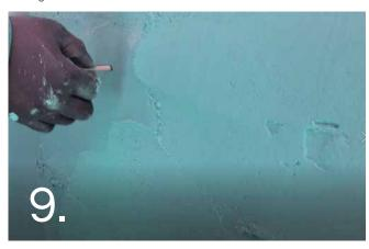
Use a gauge to check the thickness of the BeadCrete. A thin nail can be used marked at 8mm with some masking tape.
