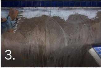
Dirty surfaces, particularly on the floor, should be pre-dampened and then acid-washed and vigorously brushed and flushed with plenty of clean water. NB: To ensure the neutralization of the surface it is essential that the surface is washed with a solution made up of a 1:10 ratio of Sodium bicarbonate and water and then rinsed with clean water again.
