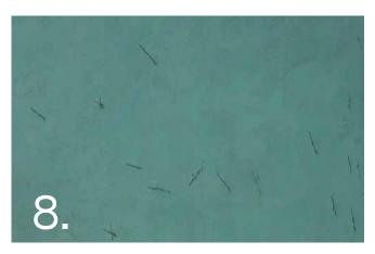
Be sure to keep an eye out for bubbles below the surface. These need to be cut with the trowel and re-floated to remove the air.
