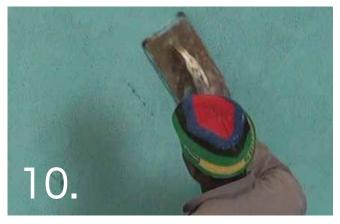
Once the BeadCrete has started to set, weather dependent, the surface needs to be sponge floated (Rhinolite floats) to flatten the surface.
