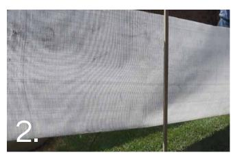
Set up sun and wind barriers prior to the application of BeadCrete to avoid premature moisture loss and plaster shrinkage.
