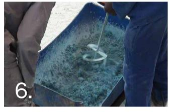
DO NOT mix inside the pool. Mix in suitably sized plastic drums. Mechanical mixers must be used and must be clean. Maximum water content per 20ka of BeadCrete must not exceed 3-4 litres. Keep mix batches as consistent as possible, DO NOT use a hose pipe, water must be measured out.
