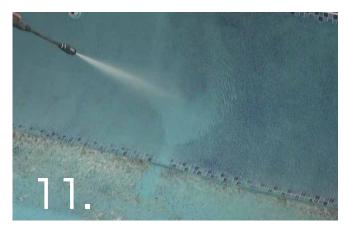
Once the surface is slightly firm, a high pressure washer is then used to wash the plaster off the beads. DO NOT spray too close as this will damage the  $\,$ plaster. Only allow the mist to gently wash the surface. Once sprayed, steel float again.
