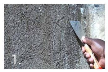
Gunite, hand-packed concrete or scratch coat cement plaster that has cured for at least 28 days. All surfaces should be true in plane, hard and slightly rough (i.e scratch plaster type finish) to ensure a good mechanical key.
