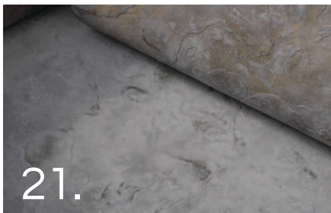
Remove the imprint mat carefully. Always fold the imprinting mat to the point of least resistance / suction.
