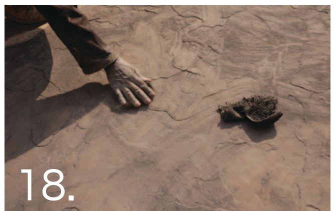
Dust Coloured Release Agent onto the smooth surface and the imprint mat. This will ensure that the mat does not stick to the surface.
