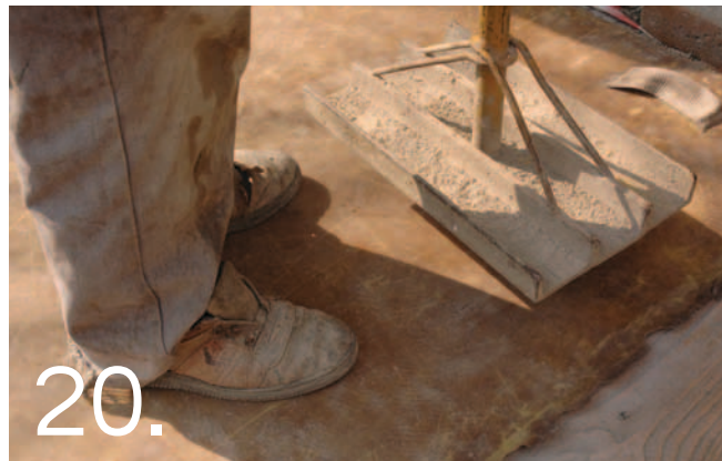
Stamp the imprint mat to transfer the design onto the surface.
