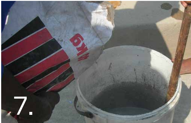
7. Mix MatCrete with enough mixing liquid to obtain a paintable consistency.
