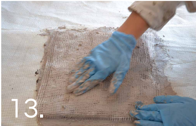
13. Use a trowel or your hands to embed the CemForce into the surface.
