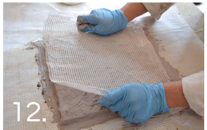
12. While still wet, place a layer of CemForce over the panel.
