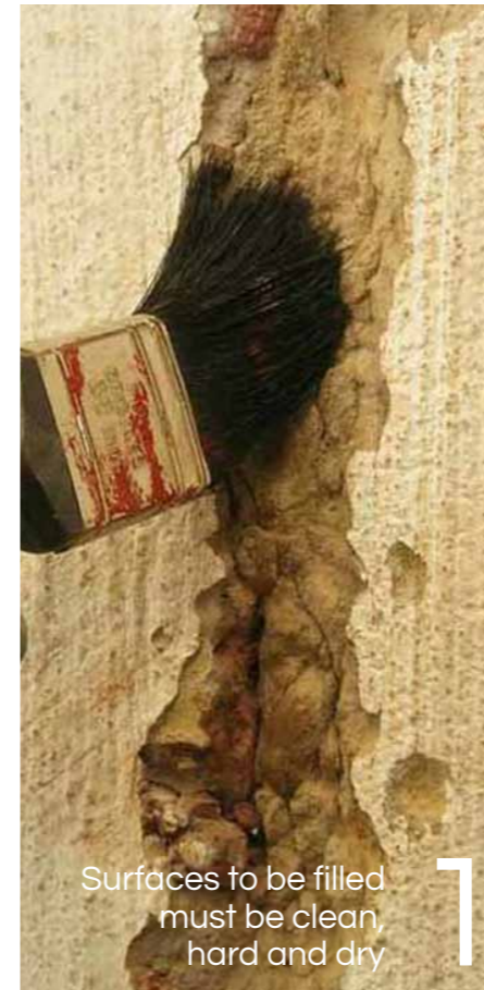
Fill cracks and holes using a paint scraper, putty knife or trowel 2
