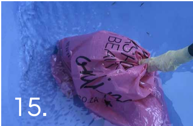
15. Commence filling the pool from the deep end. We recommend the use of a deflector on the end of the hosepipe to prevent damage to the surface. Fill the pool in one go to avoid a water ring from forming. Damp down the exposed PoolCrete every hour to prevent premature drying. Protect the plaster from staining (particularly from mud splashes) until the pool is filled.
