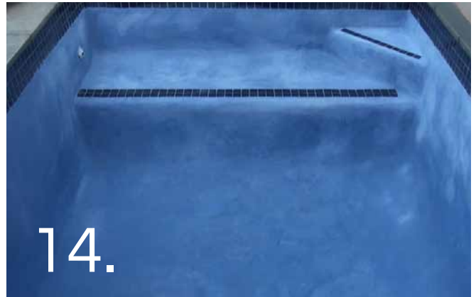
14. Filling of the pool can commence \pm 6 to 8 hours after plastering has been completed depending on ambient temperatures & relative humidity where plastering has been completed early afternoon. Where this is not the case & the plastering is completed late afternoon or early evening it is recommended that the filling process commences the morning following the application.
