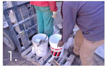
Dilute 1 part FlexBond with 4 parts water. Stir this solution very well.
