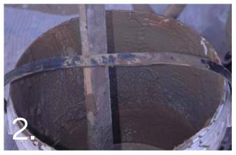
Add MatCrete to the solution until a thick paintable solution is obtained. Keep on mixing the solution to keep it thick and paintable.
