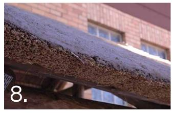
Over hanging material can be cut back once the MatCrete has dried properly (approximately 24hrs). This can be done by using a baby grinding machine fitted with a cutting disc.
