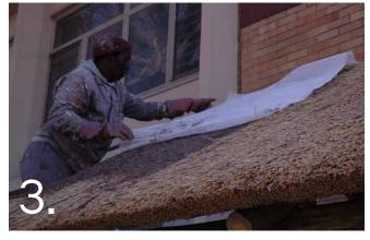
Paint a coat onto the grass working against the grain. Immediately lay the CemForce onto the wet MatCrete.
