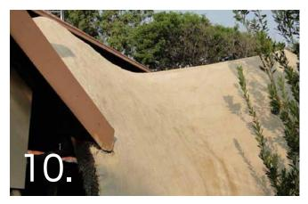
Alternatively FlexBond can be replaced with Cemcrete's CreteBond as the mixing liquid with MatCrete. This will render the MatCrete UV stable and therefore can be left as the final coat (no need for CemWash).
