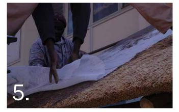
Apply another coat of MatCrete on top of the CemForce, saturating it completely.
