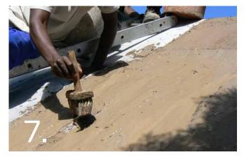
Apply a third coat of MatCrete not longer than 3 hours after the top coat had been applied. Make sure that all holes are properly filled.
