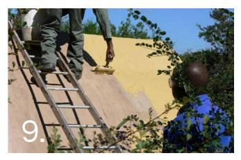
MatCrete can be coated with 1 coat of Cemcrete's CemWash (colour of choice) to obtain the desired colour of your choice. Please read the CemWash technical datasheet for application and mixing instructions.
