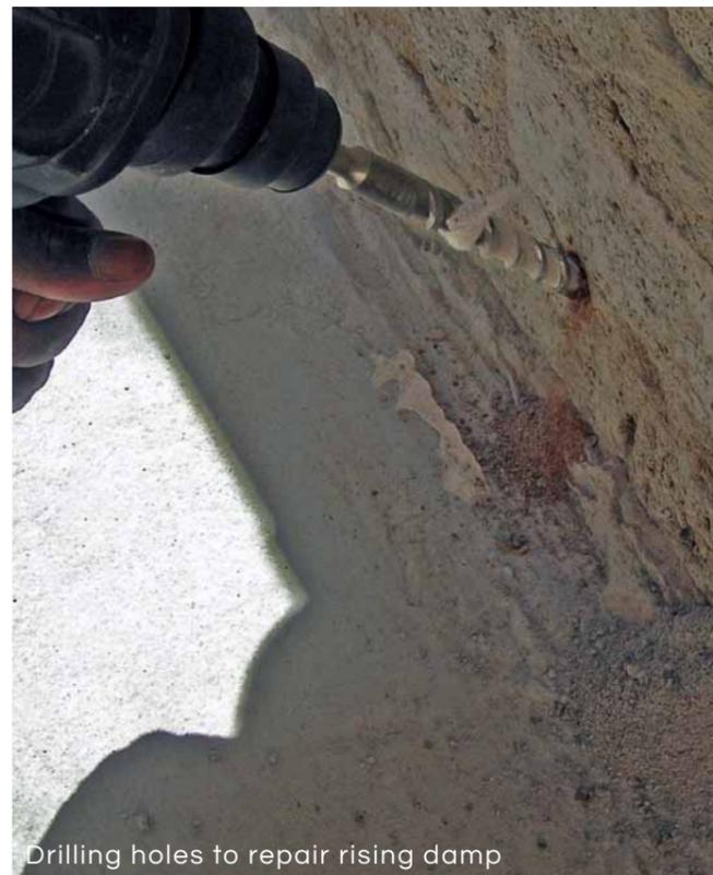
Drilling holes to repair rising damp
