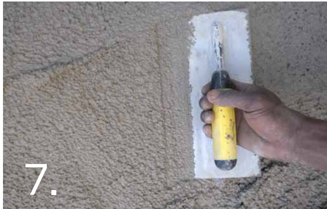
7. Apply the mixed Exposed Aggregate to a thickness of 8mm with a suitable steel trowel onto the tacky Concrete Primer to ensure a proper bond between layers.
