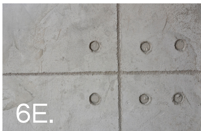
Off Shutter Finish (5mm) | Finish using a steel trowel.
