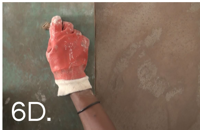
Printed Finish (5mm) | Use rubber print mats for various finishes. Can be used with Coloured Release Agent.
