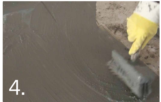
4. Apply PrimerCote slurry to small sections at a time, cover with screed mix and repeat. Do not apply too thin and do not allow to dry prior to covering with new screed mix. Immediately place screed mix onto wet slurry.
