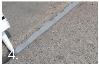
All construction, cold joints, structural joints and/or structural cracks which  $may\,be\,dynamic\,before\,and/or\,after\,the\,Exposed\,Aggregate\,application\,must$ be extended through to the surface of the Exposed Aggregate application in the form of voided joints. All voided joints including saw cuts should be filled with suitable joint filler where applicable.
