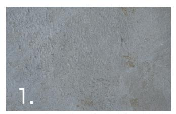
New concrete surfaces must be wood floated and fully cured for 28 days prior to application of Exposed Aggregate. The surface must be structurally sound, level, clean, dry and free from any curing agents, laitance and surface contamination such as dust, dirt, waxes, oils, old adhesives, grease, sealants, weak cement screeds etc. which may interfere with adhesion.
