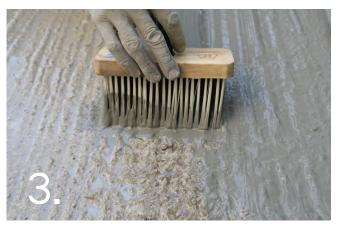
Application over moving joints or cracks can result in cracking and delamination. Cemcrete's PrimerCote mixed with FlexBond (diluted 1:3 with water) to a stiff paste can be used to patch. The surface, once repaired, must be primed with PrimerCote as per its datasheet, and leave to dry overnight.
