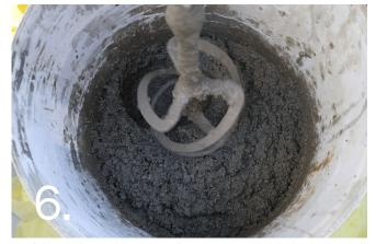
The following day apply one coat of Concrete Primer and when tacky apply the Exposed Aggregate, add 2 to 2.4 litres of clean potable water to a 20kg bag of Exposed Aggregate. Mix thoroughly using a mechanical mixer, until a uniform consistency is achieved.
