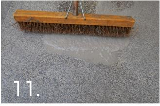
Leave the floor covered with plastic for at least 3 days in summer and 4 to 5 days in winter, the area should be washed using a portable high-pressure water washer with a wide slit nozzle and assisted with a fine wire or nylon brush or broom. This will assist in the exposure of the decorative stones.
