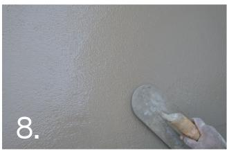
Ensure the Exposed Aggregate is floated level with the guide strips using a straight edge and then steel floated smooth. Only mix enough material to cover each panel floated flush to the guide strips.
