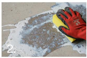
All holes and damaged areas must be repaired prior to the application of Exposed Aggregate. It is suggested to first prime shallow holes with Concrete Primer prior to patching. For larger holes use a suitable repair mortar.
