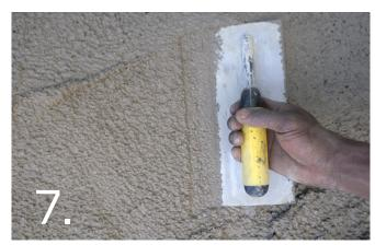
Apply the mixed Exposed Aggregate to a thickness of 8mm with a suitable steel trowel onto the tacky Concrete Primer to ensure a proper bond between lavers.
