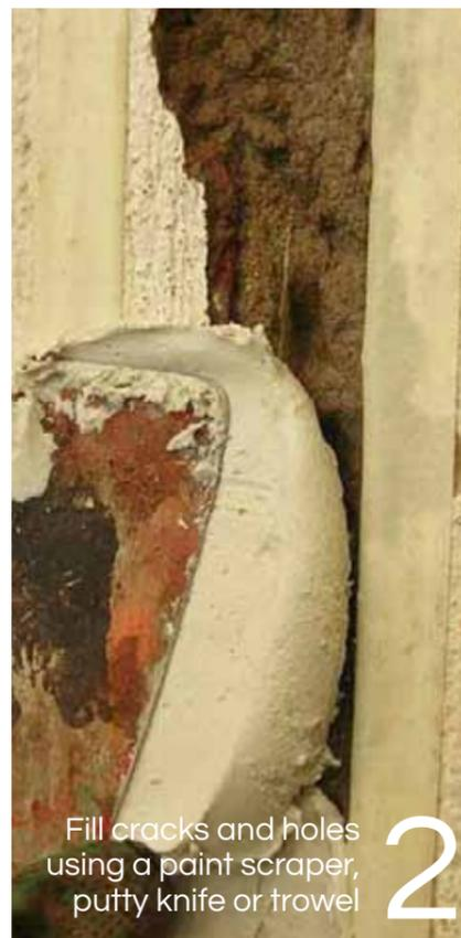
Fill cracks and holes using a paint scraper, putty knife or trowel
