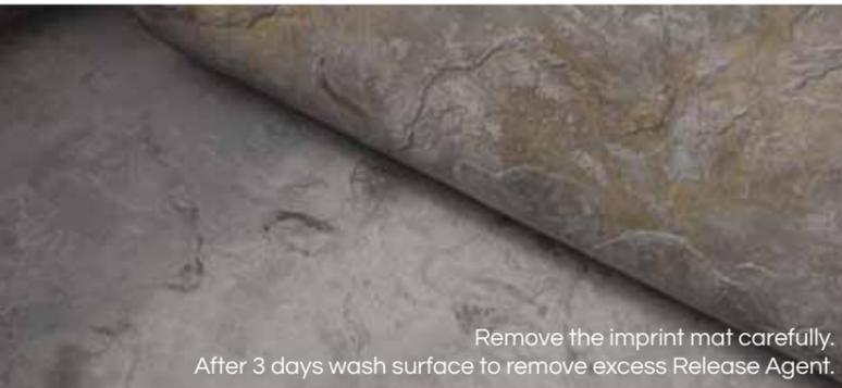
Remove the imprint mat carefully. After 3 days wash surface to remove excess Release Agent.
