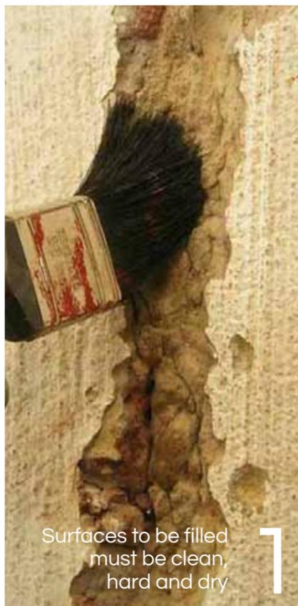
Surfaces to be filled must be clean, hard and dry
