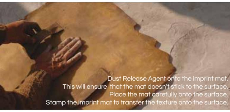
Dust Release Agent onto the imprint mat. This will ensure that the mat doesn't stick to the surface. Place the mat carefully onto the surface. Stamp the imprint mat to transfer the texture onto the surface.
