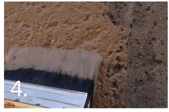
Allow the first coat to dry for 24 hours. Mist spray first twice during the day following the day of application. Once the first coat has dried, apply the second coat mixed with clean water only. Use a large paintbrush (NOT a lime wash brush or roller). Mist spray the second coat twice during the day following the day of application and allow to cure for 24 hours. It is recommended for darker colours that the final coat be cured for at least 4 days.
