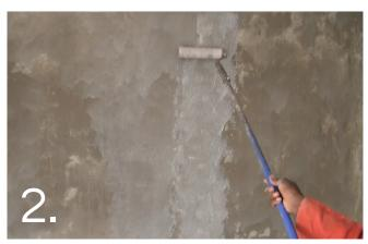
Prime wall prior to application with 2 coats of CemBond / water solution (diluted 1 part CemBond with 3 parts water).
