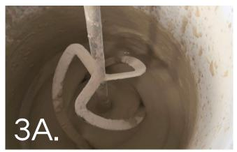
To 3 volumes CemCote stir in thoroughly 1 volume CemBond / water solution (diluted 1 part CemBond with 3 parts water) until a smooth paste is
