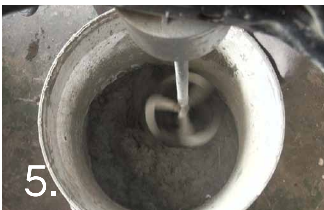
5. Leave mixture for 5 minutes before remixing and applying. Use all mixed material within 30 minutes. Half batches may be mixed for convenience. The addition of additives such as plasticizers, pigments, accelerators, etc is not recommended under any circumstance.
