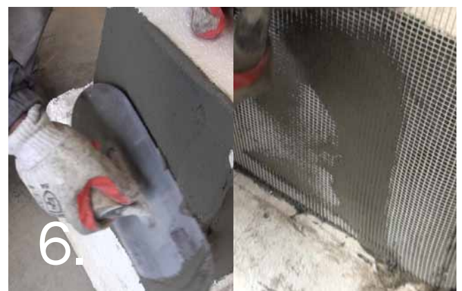
6. Apply BaseCoat Paste to a uniform thickness of about 2mm using a steel trowel. Immediately press the Glass Fibre Mesh into the wet BaseCoat Paste / cement mix.
