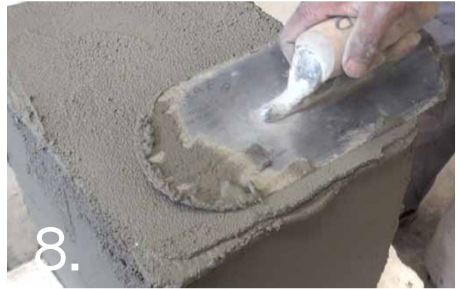
Add a final coat of BaseCoat Paste / cement mix to cover the mesh completely. Continue this process until all sides are coated with BaseCoat Paste / cement mix, Glass Fibre Mesh, secured with staples / wires, & finished with a final coat of BaseCoat Paste / cement mix.
