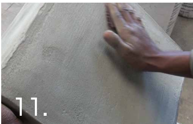
Sand the object to remove any sharp or high spots using 120 grit Abrinet sand paper. Remove all dust leaving a clean smooth surface.
