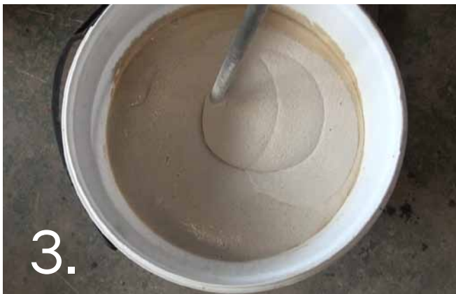
3. Premix the BaseCoat paste with clean water at a ratio of 5:1.
