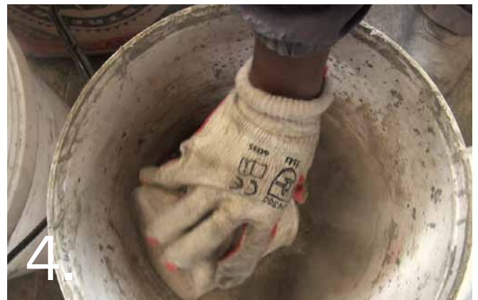
4. While stirring the BaseCoat Paste continuously, slowly add cement at a ratio of 1:1. Small amount of water can be added to obtain desired consistency.
