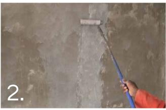
Prime wall prior to application with 2 coats of CemBond / water solution (diluted 1 part CemBond with 3 parts water). Apply the CemCote the day after
