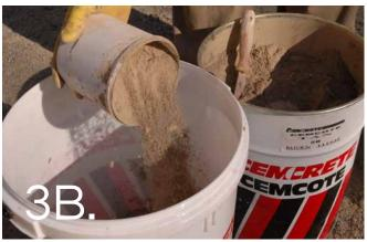
Add 1 further volume of the CemBond / water solution, mix to a paint consistency and apply within 30 minutes.
