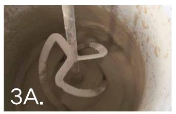
To 3 volumes CemCote stir in thoroughly 1 volume CemBond / water solution (diluted 1 part CemBond with 3 parts water) until a smooth paste is formed.
