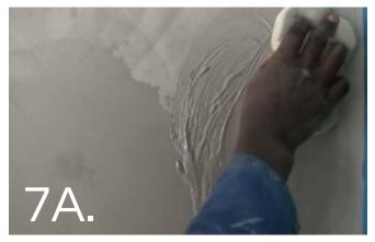
Apply the second coat and any additional coats as needed (max 0.8mm per coat), in the same manner as the first coat, until a smooth finish is achieved. First with a sponge and then...
