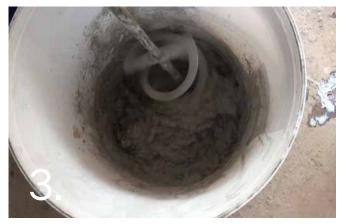
To 1 volume FlexBond / water solution (diluted 1 part FlexBond to 4 parts water), slowly add 3 volumes of CemCote powder and mix mechanically slowly until a workable plaster consistency is achieved. Do not mix manually. NOTE: For exterior use, replace the FlexBond with CreteBond. Dilution ratios stay the same as for FlexBond
