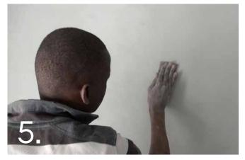
When the first coat of CemCote is dry (but within 24 hours), sand lightly by hand, in a circular motion, with 120 grit Abranet sandpaper. Always use a sanding block when sanding.
