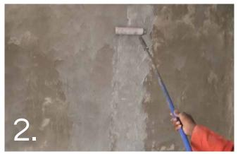
Prime wall prior to application with two coats of Cemcrete's FlexBond/water solution (diluted 1 part FlexBond to 4 parts water). Apply the CemCote the day after primina.
