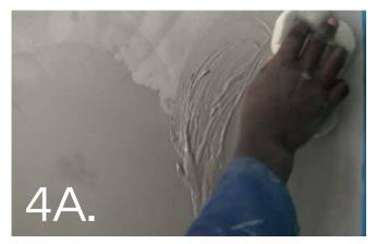
Using a firm sponge rub the first layer thinly onto the surface, follow this method small sections of the wall at a time...
