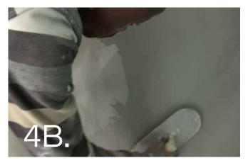
...then while still wet smooth the surface using a rounded pool trowel. Then sponge the next section and repeat the process. Each layer applied must not exceed a depth of 0.8mm even if high spots remain exposed.
