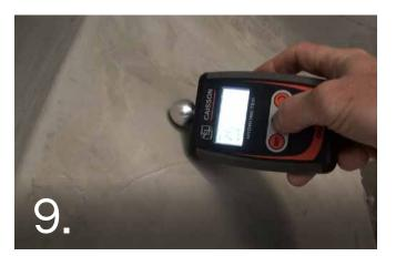
Remove all dust and protect the wall until ready for sealing. The moisture in the wall must be less than 5% before sealing.
