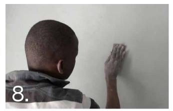
Once the final coat of CemCote is dry (but within 24 hours after the application), sand lightly with 240 grit Abranet sandpaper in a circular motion, to not leave any sanding marks and ridges on the surface. Always use a sanding block when sanding.
