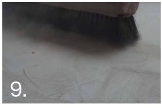
Remove all dust and protect the floor until ready for sealing. The moisture in the floor must be less than 5% before sealing.
