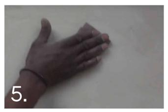
As soon as the first layer is dry, marks left by uneven trowelling should be removed by sanding by hand within 24 hours after application. Sand lightly in a circular motion using 120 grit Abranet sandpaper.
