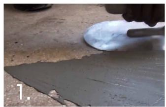
Prepare the concrete base / screed as required. Refer to product datasheet for correct procedure. Cemcrete's PrimerCote or a suitable self-leveller can be used if required. Sand high / rough spots. Substrate must attain a moisture level below 5% before the application of CreteCote.
