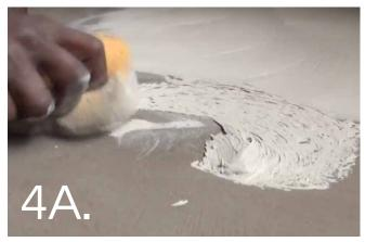
Ensure the prepared surface is cool and protected from wind, sun and other elements. Using a firm sponge rub on the first layer of CreteCote thinly onto the surface, then...
