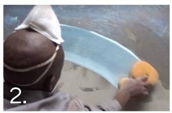
Apply two coats of Cemcrete's Concrete Primer with a sponge. A third coat may be required if the floor is very porous. Apply each coat perpendicular to the previous. Allow each coat to dry before applying the next coat. Allow to dry for 24 hours before applying CreteCote.
