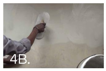
... while within arm's length, smooth the surface using a rounded pool trowel, until a smooth finish is achieved. Each layer applied must not exceed a depth of 0.8mm even if high spots remain exposed. Work small areas at close range, always maintaining a wet edge.
