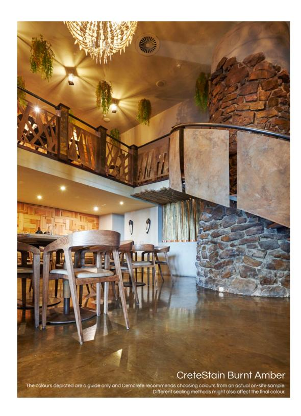
A reactive mixture containing special chemicals which reacts with the OPC (Ordinary Portland Cement) to stain & colour the surface. It produces & enhances mottling of the surface it is applied to.
