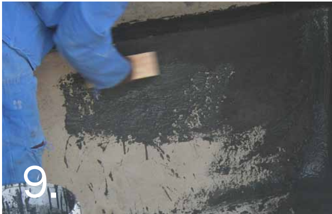
9. Apply first coat of MatCrete evenly over the entire structure using a block brush. Place a layer of CemForce over the wet MatCrete, making sure to overlap each joining piece by at least 10cm.
