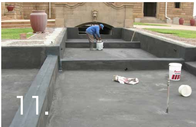
11. Apply a second coat of MatCrete once the first coat has set. This must be done on the same day. A second layer of CemForce may be applied if required. This second layer should be placed perpendicular to the first layer. Follow with a final coat of MatCrete.
