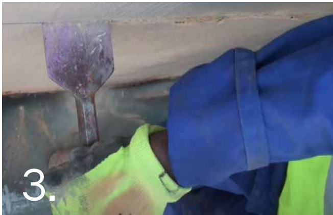
Cut back to brick using an angle grinder or chisel.
