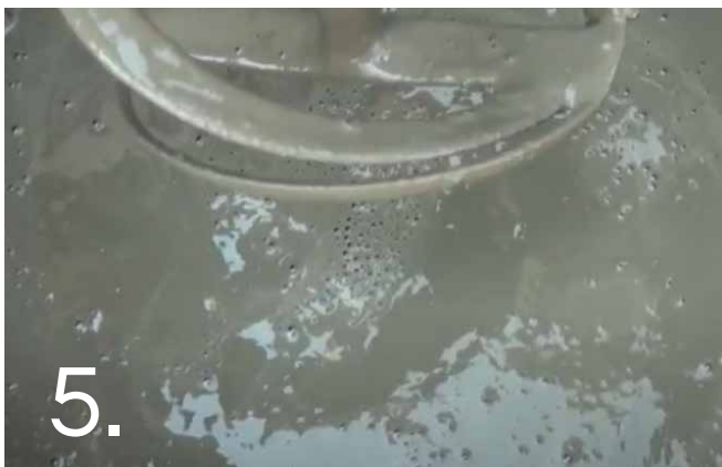
Mix 1 volume of water to 2 volumes of Permastop to a paintable consistency. Use all mixed material within 20 minutes. Do not add water to mixed material to restore workability.
