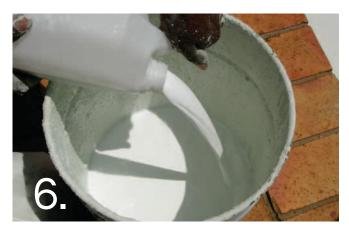
Remove contents of drum. The drum will be used as the mixing vessel. Pour the liquid from the plastic bottle into the drum. Slowly pour in the powder from the plastic bag while stirring continuously to obtain a creamy consistency.
