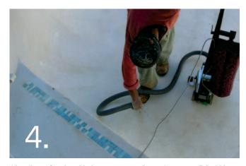
When the surface has dried, use a vacuum cleaner to remove all dust & loose material from the surface. Dust or debris will prevent proper bonding of the Pool Coating.
