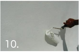
Apply the second coat using vertical strokes. A lambs-wool roller may be used. Mix 1L of Cemcrete's FlexBond with 4L of water  $\vartheta$  keep this solution on hand to mix with Pool Coating (no more than 30ml at a time) to maintain a paintable consistency during warmer temperatures.
