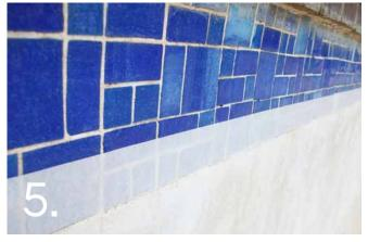
It is important to mask all pipes, weirs and mosaics etc. Masking must be removed on the same day after the Pool Coating is touch dry.
