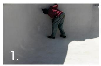
Clean the mosaics prior to emptying the pool. Remove all calcium scale using sandpaper & a paint scraper. If there is any algae, dilute 4 cups of granular chlorine in a 10L bucket of warm water  $\vartheta$  apply to the surface. Leave for 24 hours 8 then wire brush and flush off with clean water. Make sure that all crack & plaster repairs is completed & cured prior to acid wash.
