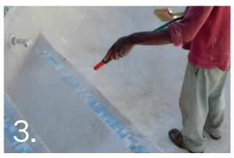
Flush clean with plenty of water. It is important to ensure that there is none of the acid wash solution left on the surface. Neutralize the plaster surface by brushing the pool surface using a solution made up of 1 cup of sodium bicarbonate and 5 litres of water. Rinse with clean water and allow to dry.
