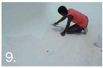
Start at the deep end & paint the walls first & then the floor. Do not patch. Leave the 1st coat to dry completely (a minimum of 3 hours). Both coats to be applied on the same day.
