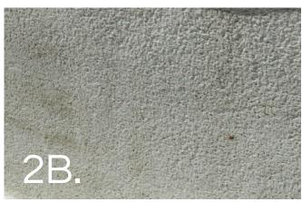
The surface must be as rough as 60grit sandpaper and free of calcium carbonate. If not, repeat the acid wash process until this is achieved. The proper cleaning and roughness of the surface is critical to ensure a good
