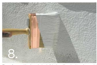
The surface must be damp, but not glistening with water. Use a large paint brush to apply the 1st coat in horizontal strokes. Finish with the tip of the brush to minimise brush marks. A wet edge must be maintained throughout the coating of the pool for both coats.
