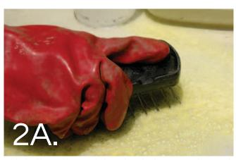
Mix hydrochloric acid & water (1:3) in a plastic bucket. Wearing gloves, apply to the surface using a block brush. Let the solution fizz for at least 5 min  $\theta$  then scrub vigorously with a stiff wire brush.
