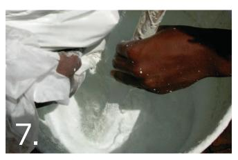
Very small amounts of FlexBond/water solution (1:4) may be added. Do not over-thin the mixture. Mixed material must be used within an hour. If a longer time is anticipated, split the packs and mix smaller batches.
