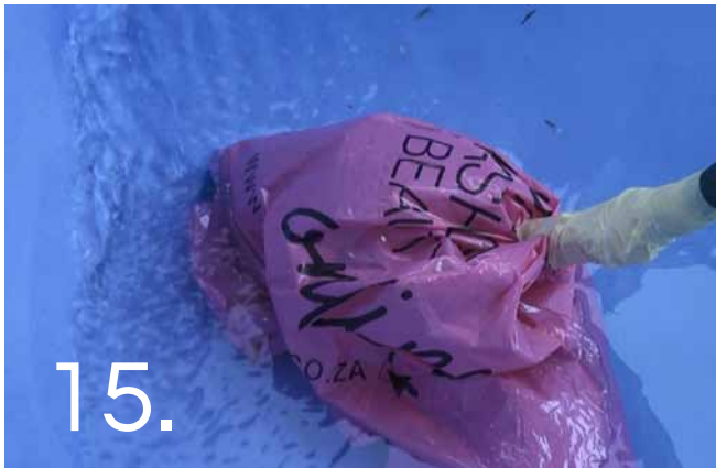
15. Commence filling the pool from the deep end. We recommend the use of a deflector on the end of the hosepipe to prevent damage to the surface. Fill the pool in one go to avoid a water ring from forming. Damp down the exposed PoolCrete every hour to prevent premature drying. Protect the plaster from staining (particularly from mud splashes) until the pool is filled.
