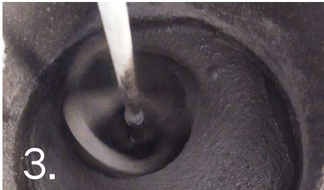
3. Mechanically mix 3 parts RenoCrete to 1 part water.
