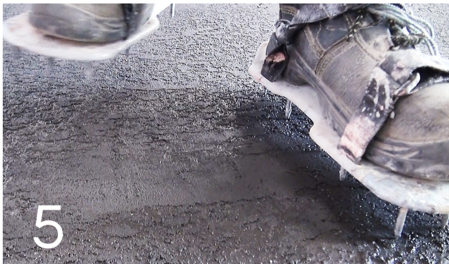
5. A team member in spiked shoes will follow the sprayer (during third coat) and...
