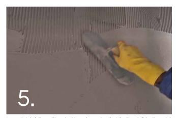
Immediately follow with a steel trowel ensuring that the lines left by the notch
