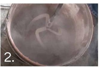
Mix 1 volume clean water to 4 volumes of RenoCrete and mix thoroughly using a mechanical mixer.
