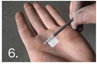
At this stage check the depth of the RenoCrete using a 3mm gauge, and either add or remove product as required. A 3mm gauge can be made using a nail and masking tape.
