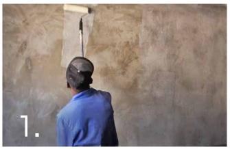
The plaster should be cured for at least 21 days before RenoCrete is applied. Prime the plaster with a solution made up of 1 part CemBond and 5 parts water. Apply two coats of this solution and overcoat when first coat is dry. Apply RenoCrete the next day.
