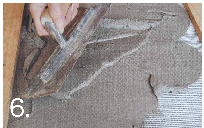
6. Use a trowel to spread evenly.
