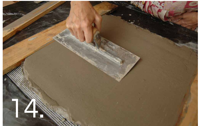
14. Use a trowel to smooth the surface and remove lines.
