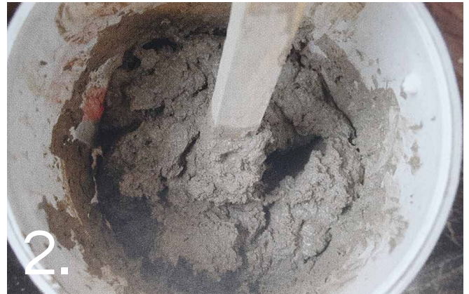
2. Mix to a paste with no slump. It may be necessary to add extra mixing liquid. The mix should not be too stiff.
