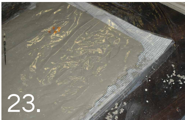
23. When the design is completed, cover with plastic and leave overnight. Remember to trim the edges. Replace plastic and spray with water 3 times during the next day. Leave overnight. Remove plastic and leave to dry for at least 3 days before sealing.
