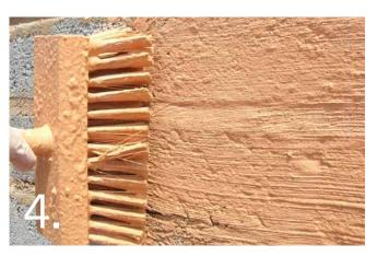
Wet the brush or broom and shake off excess water. Dip the brush in the StippleCrete mixture and liberally apply to the wall from bottom to top. Make sure all small holes and indentations are filled. If further texture is required, use block brush to stipple.
