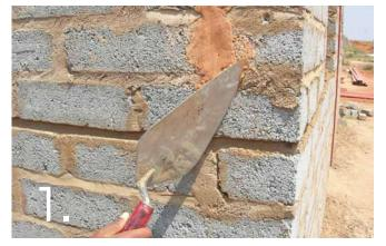
All applicable surfaces to be structurally sound and free from grease, oil, wax, wall paper glue, dust or anything that might interfere with adhesion. Remove dust and loose defective paint if any. Important that the wall is also flat and smooth. Use a stiff mix to fill imperfections, cracks and holes in the brickwork ensuring that it is finished flush with the surrounding surface.
