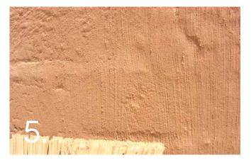
Work from one architectural feature to another keeping a wet edge in material to prevent unsightly dry joints. Do not come back to patch. Clean splashes and over-brushing at the end of each day.
