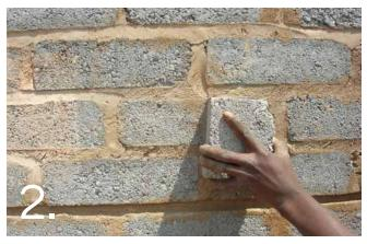
Allow this to dry and then using a rubbing brick rub the entire surface so as to remove all high spots before applying StippleCrete. Surfaces should be primed with 2 coats of a solution of 1 volume CemBond, and 5 volumes of water
