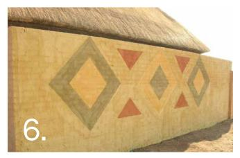
Following the day of application, cure by wetting all completed work 3 times during the day, to ensure hardness and durability. Always cure from bottom to top in order to avoid water run marks and colour variations.
