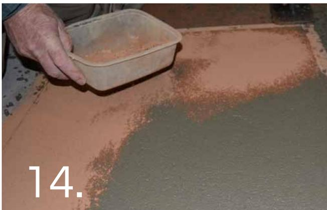
Apply Colour Hardener powder to the damp SuperScreed at a rate of 2kg/m<sup>2</sup>.
