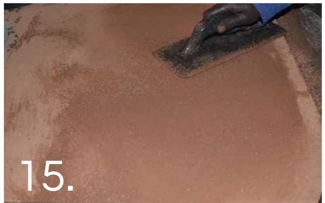
Once shaken over the surface, allow the moisture from the screed to surface, making the powder paste easy to float in. Using a wooden trowel, work the powder into the screed.
