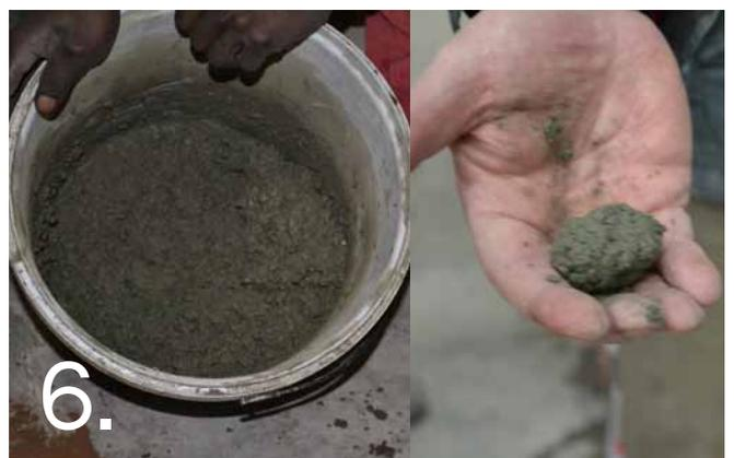
6. The consistency should be that of a damp yet firm dagga.
