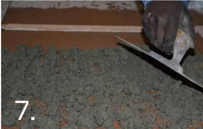
Throw some of the SuperScreed mix onto the wet PrimerCote. Using a steel trowel to evenly distribute the mix.
