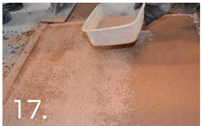
Apply a second application at a rate of 3kg/m<sup>2</sup>. Repeat steps 15 and 16.
