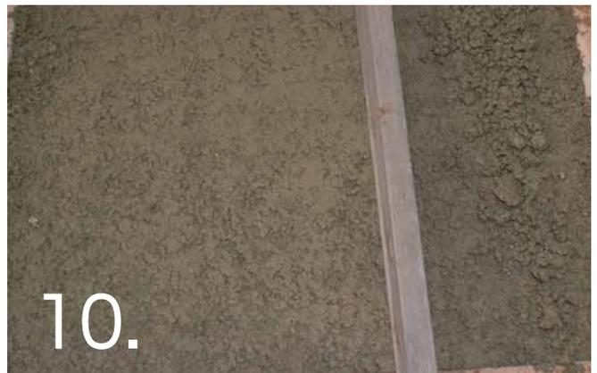
Using a straight edged rod, further level off the SuperScreed.
