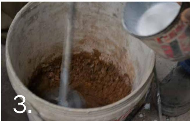
3. Thoroughly mix using a mechanical mixer.
