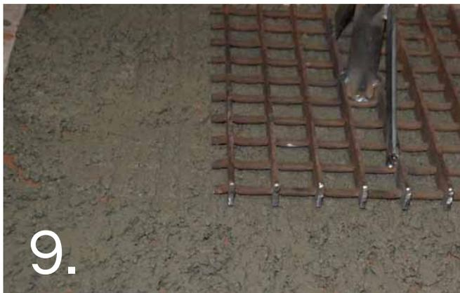
Using a steel meshed stamper, continue to compress the SuperScreed. This will allow air to be released and consistent levels to be achieved.
