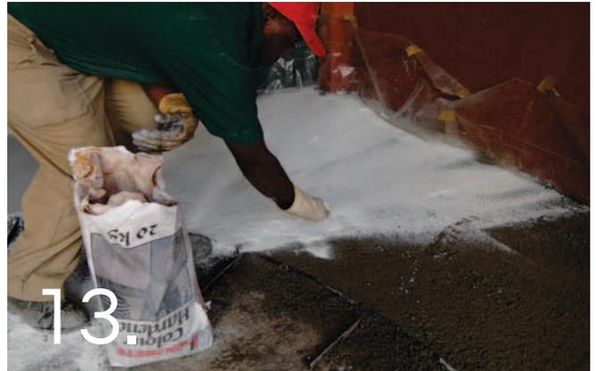
As per Colour Hardener's datasheet and step-by-step, Colour Hardener is a dry shake powder which you float into a wet screed. Application can be done by hand, or by using a container with holes in the bottom to ensure an even, consistent distribution and coverage.
