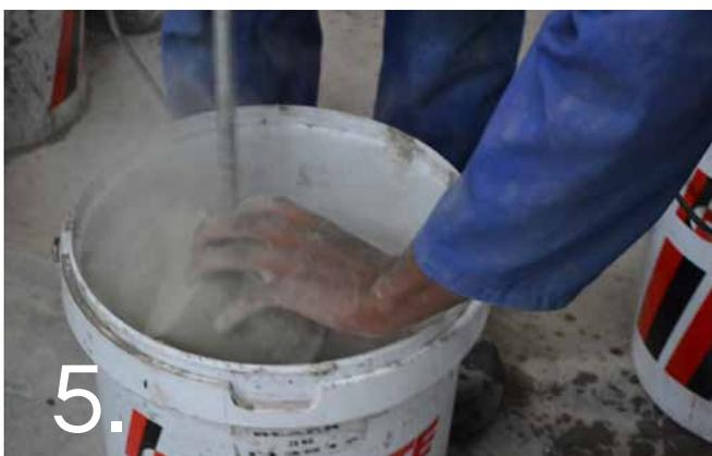
5. Mix one 40kg bag of SuperScreed powder with 5L of clean water using a mechanical mixer.
