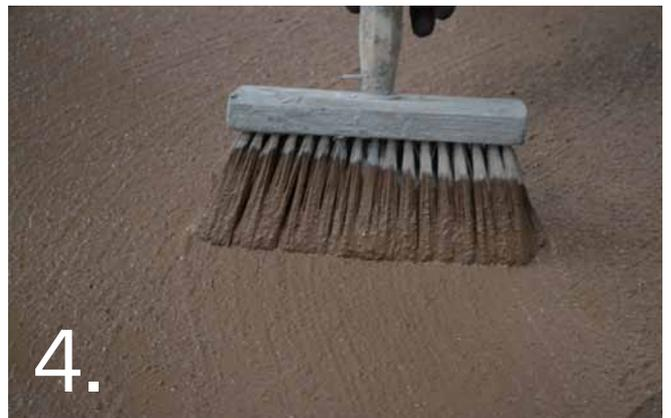
4. Using a block brush, liberally brush the PrimerCote slurry onto a clean surface.
