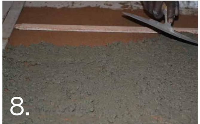
Work quickly (as the PrimerCote is painted on) apply the SuperScreed mix by trowel, compressing the mix as you go.
