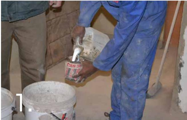
1. Dilute Cemcrete's FlexBond with water in a ratio of 1 part FlexBond and 2 parts water.
