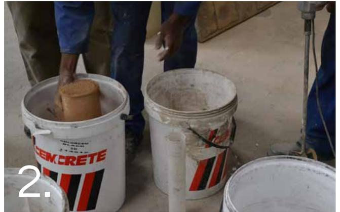
2. Combine 3 parts of the PrimerCote powder with 2 parts of the diluted FlexBond mixture.
