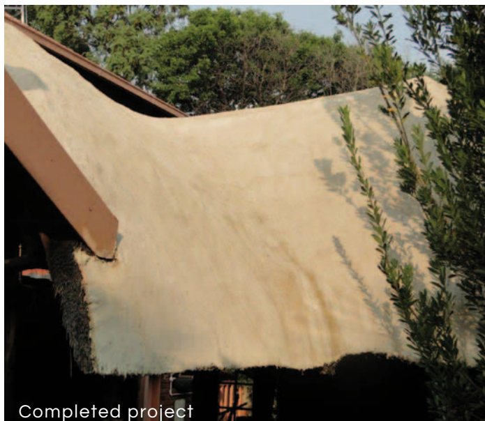
CemForce placed over thatching
