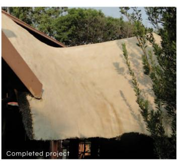
For creating a thin, reinforced, waterproof cement lining which is a low conductor of electricity & which can be applied directly onto the exterior of an new or old combed grass thatched roof. This lining is tough enough to resist mammals & birds from causing damage to the roof or entering the building.
