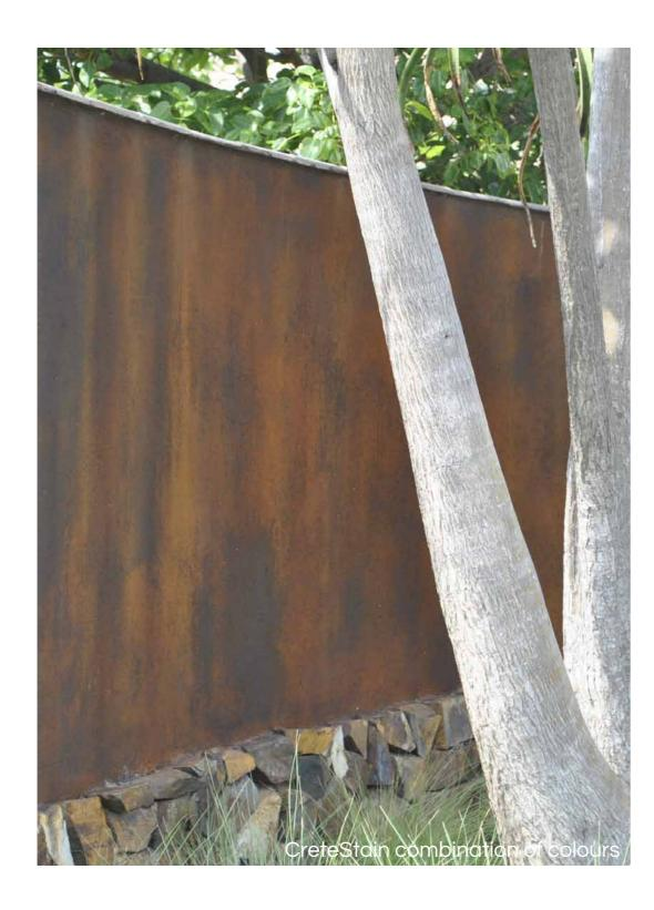
A reactive mixture containing special chemicals which reacts with the OPC (Ordinary Portland Cement) to colour the surface. It produces and enhances mottling of the surface it is applied to.
