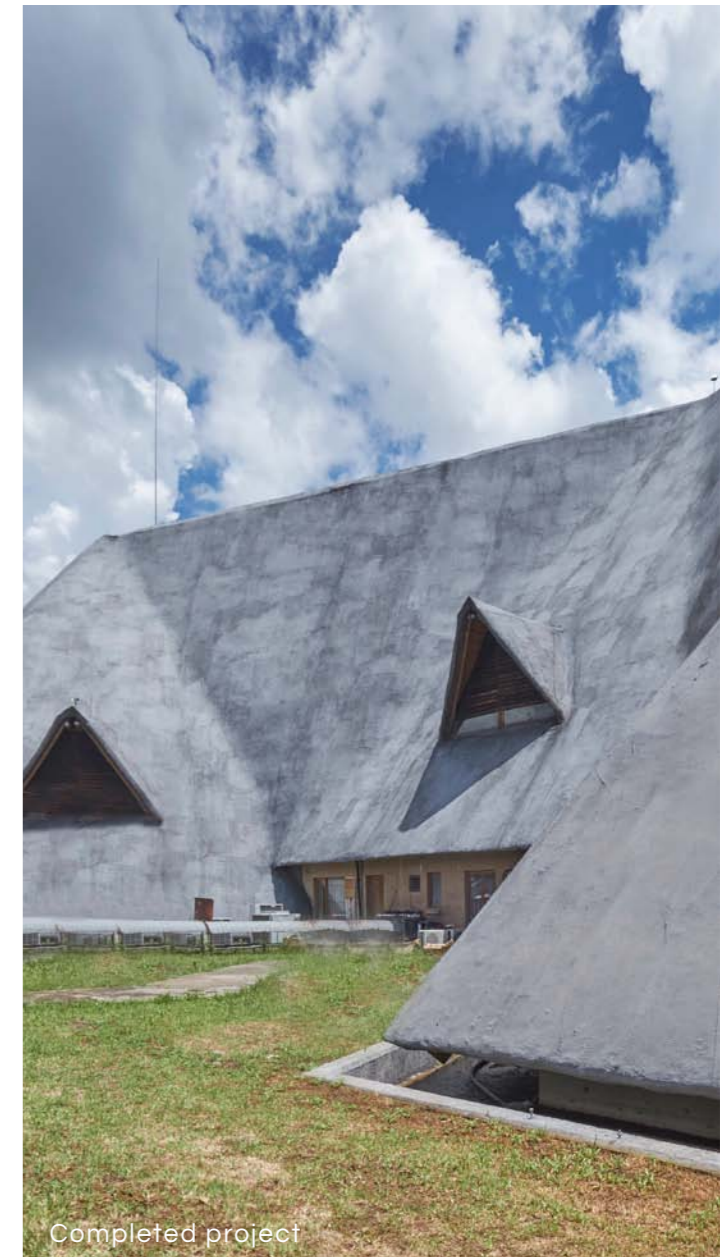
ThatchCrete system application over thatching
