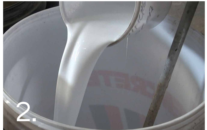
Combine 1 volume of CemBond with 5 volumes of clean water. Use this Mixing Liquid to prime the surface. Leave until the surface is tacky (usually about 10 minutes).
