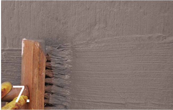
7. Optional: Apply the CemWash (Colour) at a 90° angle to the CemWash first coat grey. This will produce a "heassian" affect.
