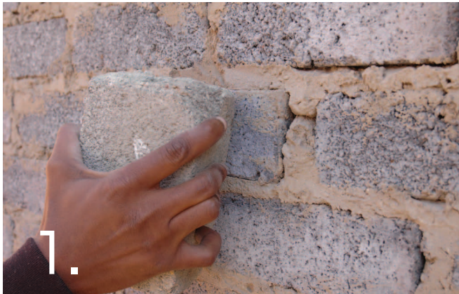
1. Remove high spots by rubbing a brick over the surface in a circular motion.
