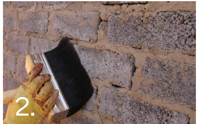
2. Remove all dust and loose material.
