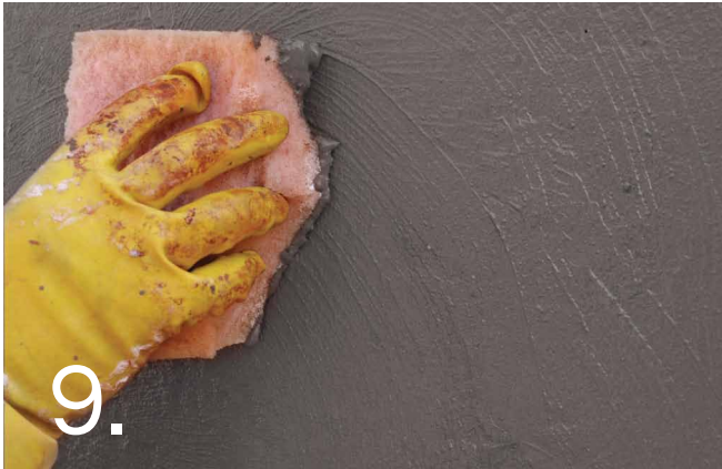
9. Optional: Finish the final CemWash coat using a damp sponge to create desired texture.
