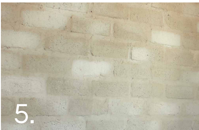
5. Mix the CemWash Colour coat in the same manner as the CemWash first coat grey. Apply with a block brush. Cure by wetting with clean water 3 times the next day from the bottom upwards. Leave to dry. Where a high level of dirt retention is expected we recommend the use of a sealer. The moisture in the substrate must be less than 5% prior to sealing.
