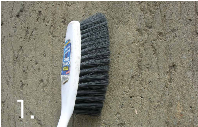
Remove all dust and loose material by brushing well.
