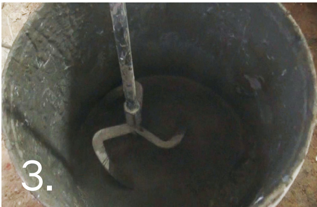
3. Mix 1 volume of FlexBond with 2 volumes of water. Use this liquid to mix 3 volumes of PrimerCote powder with 2 volumes of the liquid mix. Dampen down floor prior to applying the PrimerCote slurry to prevent rapid drying. Do not leave puddles.
