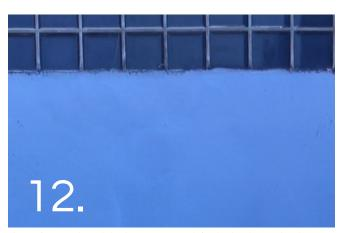
The surface can be polished to a very smooth finish when biscuit-hard. Always complete plastering in one day to avoid dry joints.
