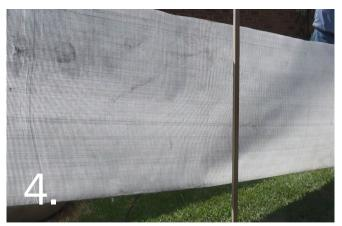
Set up sun and wind barriers prior to the application of PoolCrete to avoid premature moisture loss and plaster shrinkage.
