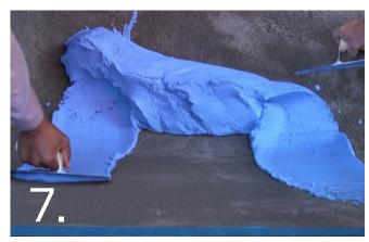
Apply PoolCrete 6mm thick with flexible rounded steel trowels. Apply the first layer, forcing the material tightly against the surface. The first layer is followed immediately by a second trowel with more material to an application not exceeding 6mm. It is easier to plaster the walls first 8 continue onto the floor.
