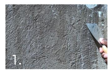
Gunite, hand-packed concrete or scratch coat cement plaster that has cured for 28 days. Must not contain blast furnace slag as this could cause mottling of the PoolCrete. All surfaces should be true in plane, hard and slightly rough (i.e. scratch plaster type finish) to form a mechanical key.
