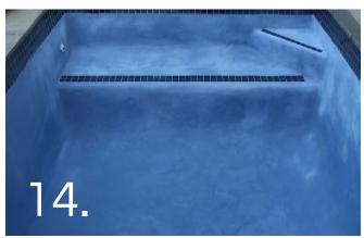
Filling of the pool can commence  $\pm 6$  to 8 hours after plastering has been completed depending on ambient temperatures & relative humidity where plastering has been completed early afternoon. Where this is not the case  $\boldsymbol{\vartheta}$ the plastering is completed late afternoon or early evening it is recommended that the filling process commences the morning following the application.
