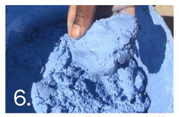
Maximum water content per 40kgs of PoolCrete must not exceed 6 to 7 litres. Mix PoolCrete with clean water to a stiff workable plaster mix (±5mm slump). The mixed plaster must look almost too stiff.
