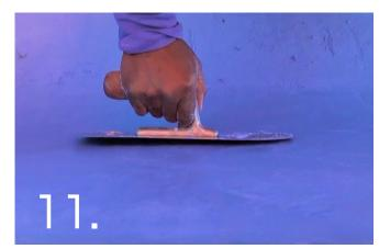
Allow to stiffen for approximately 30 min, depending on the weather, & retrowel to smooth out ridges & trowel marks. Avoid splattering additional water onto the PoolCrete surface as this will result in colour variation.
