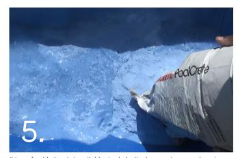
It is preferable to mix in suitably sized plastic drums using a mortar mixer or hand mixed on a board or tarpaulin outside the pool. Mixing inside the pool increases the risk of plaster discolouration, separation or debonding as a result of mix water saturating the substrate prior to plastering.
