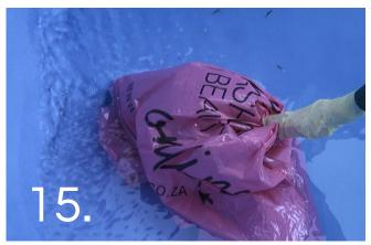
Commence filling the pool from the deep end. We recommend the use of a deflector on the end of the hosepipe to prevent damage to the surface. Fill the pool in one go to avoid a water ring from forming. Damp down the exposed PoolCrete every hour to prevent premature drying. Protect the plaster from staining (particularly from mud splashes) until the pool is filled.
