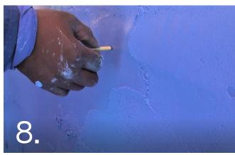
Use a 6mm gauge to check thickness (a thin nail marked at 6mm with masking tape can be used).
