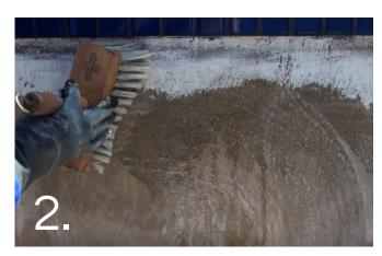
Dirty surfaces, particularly on the floor, should be pre-dampened and then acid-washed and vigorously brushed and flushed with plenty of clean water. To ensure the neutralization of the surface we recommend that the surface is washed with a solution made up of 1 cup of sodium bicarbonate to 5 litres of water and then rinsed with clean water again.
