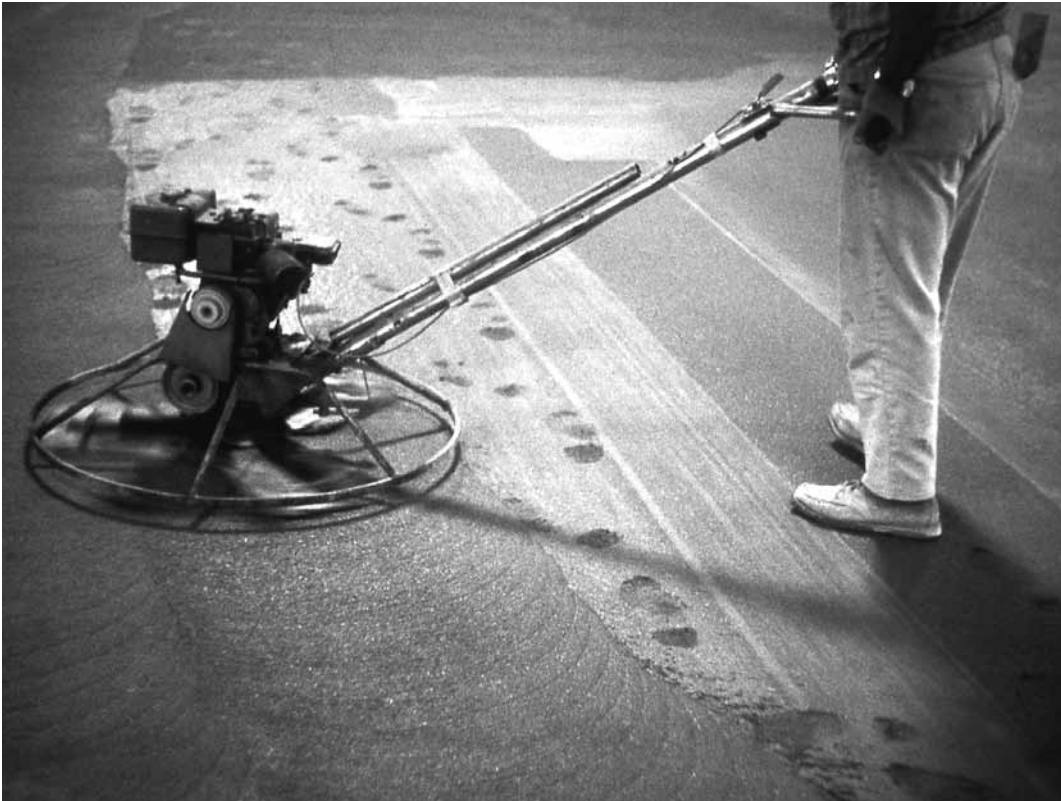
Power floating a screed.
