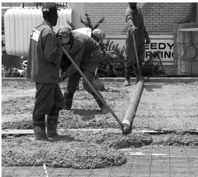
Levelling a concrete topping. Reinforcement and temporary screed battens in the foreground.
