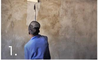
The plaster should be cured for at least 28 days before SatinCrete is applied. Prime the plaster with a solution made up of 1 part CemBond and 5 parts water. Apply two coats of this solution and overcoat when first coat is dry. Apply SatinCrete the next day.
