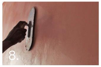
Followed immediately by smoothing with a slightly damp steel trowel. Note: Do NOT splash water onto the surface (as this will discolour the final finish), rather gently wet the steel float itself.
