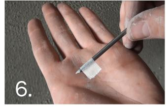
At this stage check the depth of the Satincrete using a 3mm gauge, and either add or remove product as required. A 3mm gauge can be made using a nail and masking tape.
