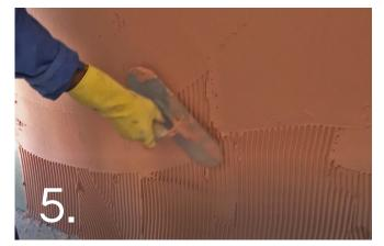
Immediately follow with a steel trowel ensuring that the lines left by the notch trowel have been flattened.
