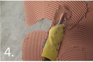
Using a 6mm steel notch trowel, apply the first layer forcing the material tightly against the surface (similar to tile glue).
